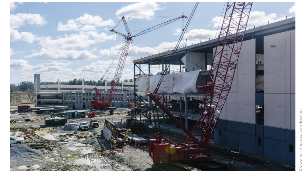
Above: At the Howard County Circuit Courthouse project, the team is installing the structure's precast and punch window façade. Left: The team recently live-streamed a joint sealant pull test to accommodate virtual participation from key stakeholders.
