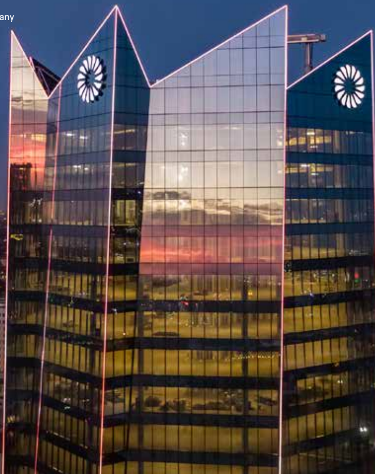
Frost Tower San Antonio, TX Photo by: White Cloud Drones
