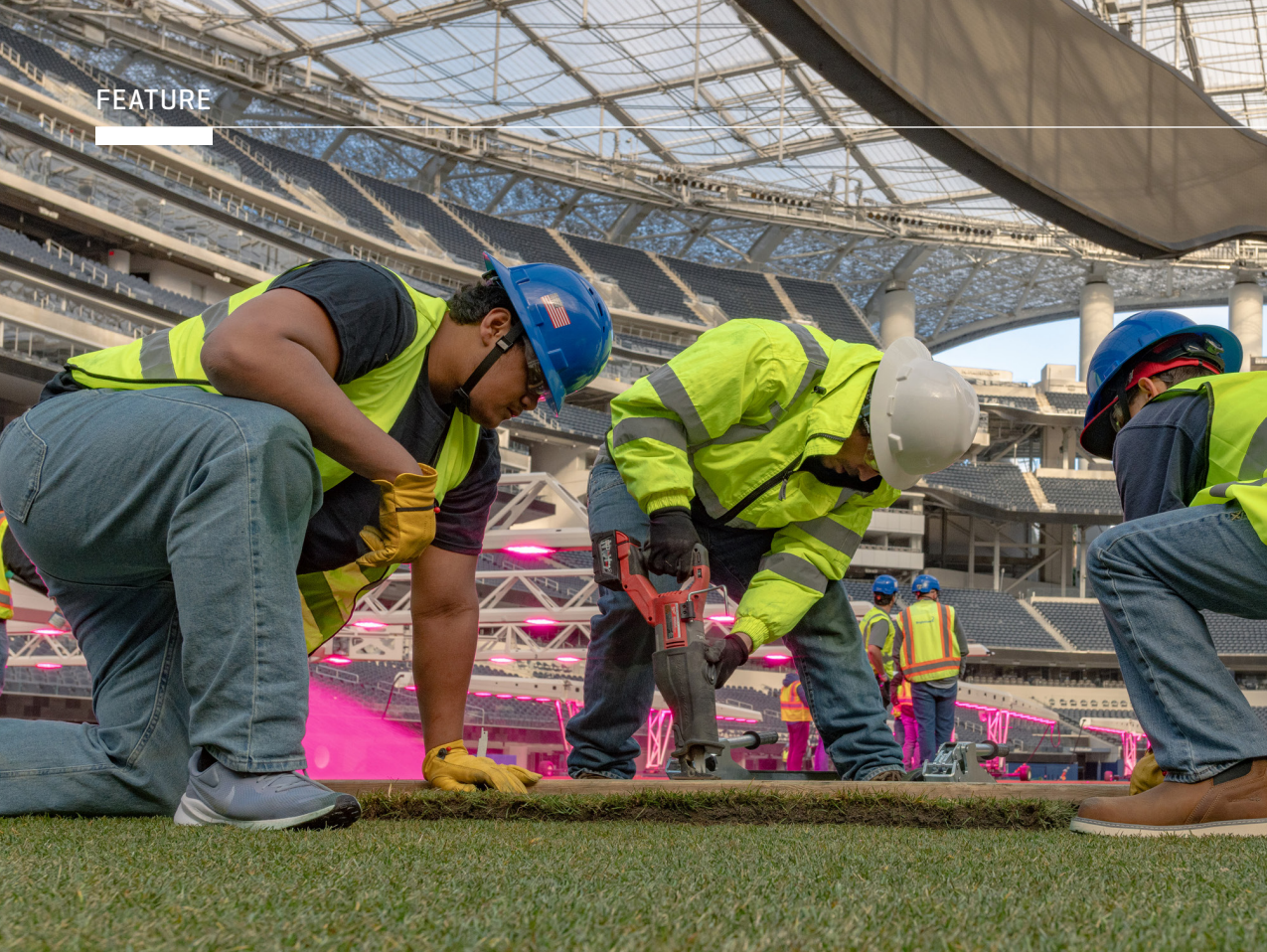
Left: Crews install the sod at SoFi Stadium, which was grown nearly a year in advance at a sod farm in Washington.
