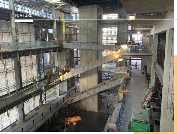
The structural renovation included removing large portions of four floors between levels one through six and replacing the south and east façades.
