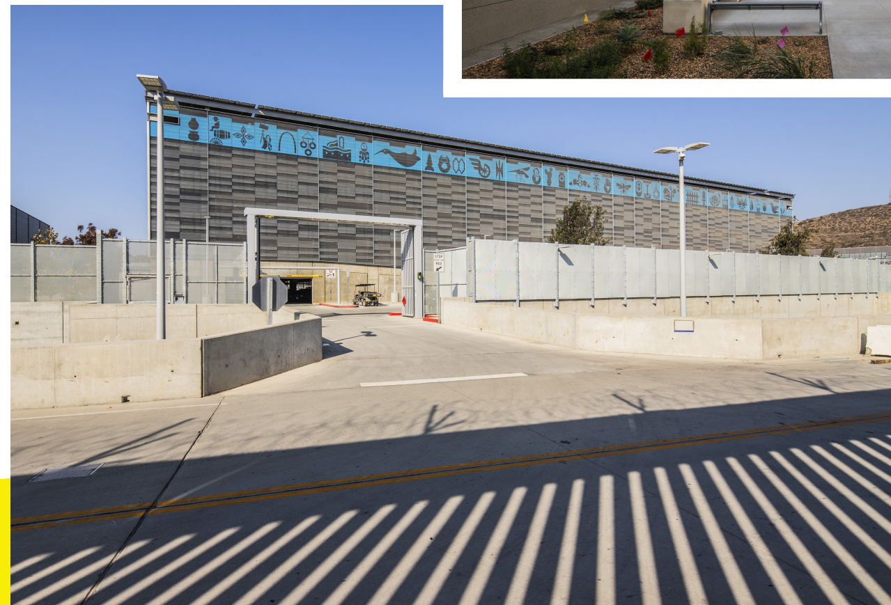
SYLPOE is on track to achieve a LEED Platinum rating. Above: Drought resistant native plantings in bio-retention and filtration areas is one sustainable water management feature on the campus. Left: The façade of the parking garage is clad in a perforated horizontal metal panel system, which allows for open-air ventilation, visual seclusion, and shade. The façade also integrates a band of graphic symbols as a historical aspect and contextual narrative of the site.
