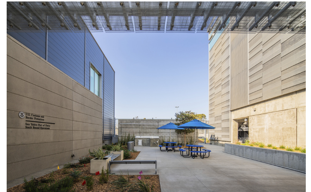
SYLPOE is on track to achieve a LEED Platinum rating. Above: Drought resistant native plantings in bio-retention and filtration areas is one sustainable water management feature on the campus. Left: The façade of the parking garage is clad in a perforated horizontal metal panel system, which allows for open-air ventilation, visual seclusion, and shade. The façade also integrates a band of graphic symbols as a historical aspect and contextual narrative of the site.
