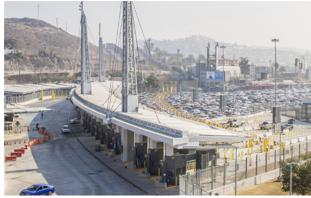
A 750-foot-long catenary-suspended canopy above the vehicle inspection booths affords uninterrupted sightlines and much-needed illumination for officers as they perform inspections (above). It also serves as a canvas for an art installation comprised of LED lights spanning the length of the southern side of the canopy (right).
