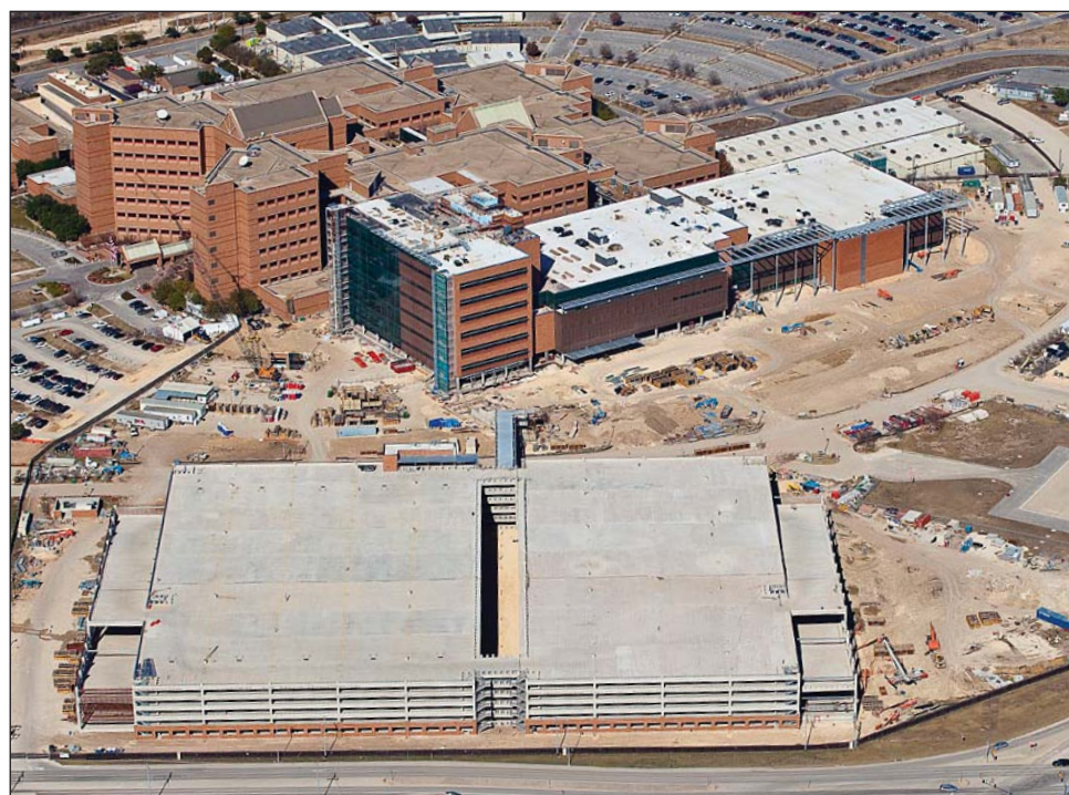
Construction continues at SAMMC-North, San Antonio (Photo by Eric Richter)
