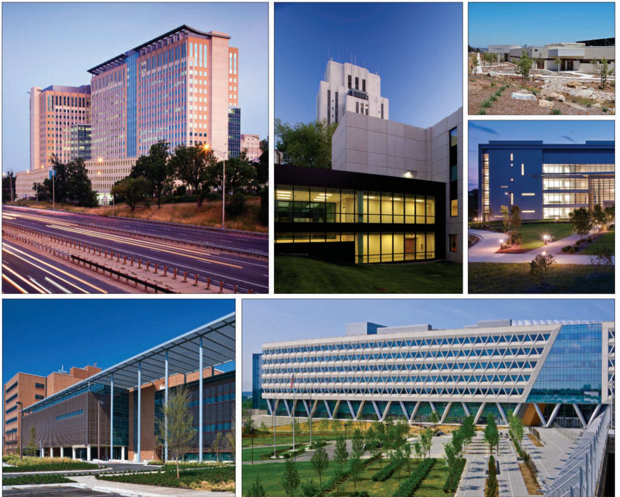
Clark's BRAC projects. Top Row (L to R): DoD/BRAC 133, Alexandria, Va.; Walter Reed National Military Medical Center, Bethesda, Md.; Joint Regional Correctional Facility Southwest, San Diego; and Air National Guard Headquarters and Readiness Center, Camp Springs, Md.; Bottom Row (L to R): San Antonio Military Medical Center, San Antonio; and NGA Campus East, Fort Belvoir, Va.
