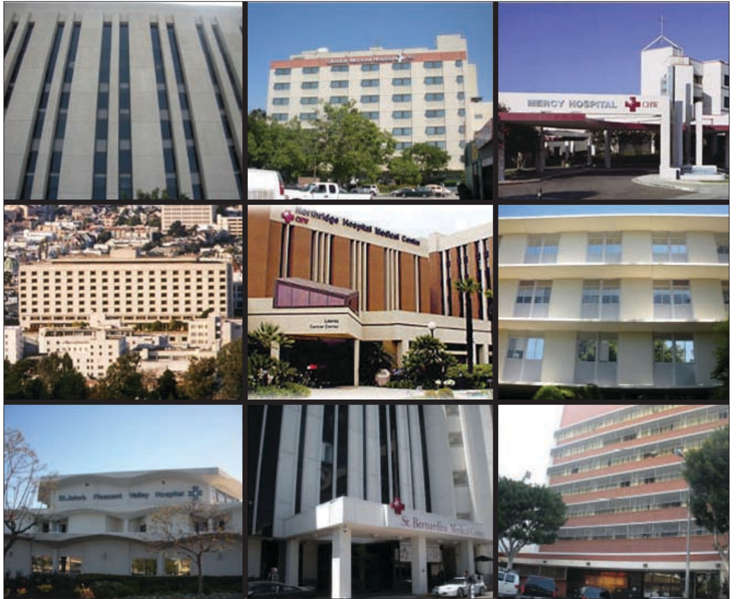
Nine Catholic Healthcare West facilities are slated for seismic retrofits.
