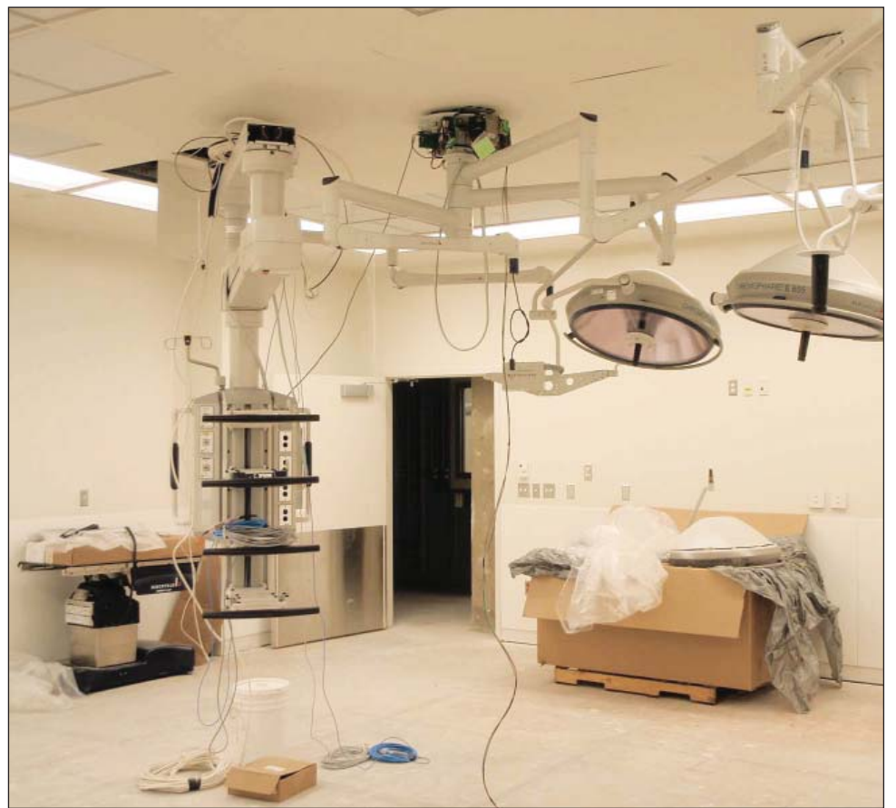
Operating room mock-up under construction at the New Clinical Building.
