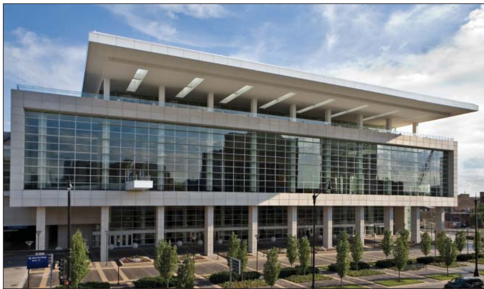
McCormick Place West Expansion, Chicago (Photo courtesy of REALVIEWS by Cesar Russ)
