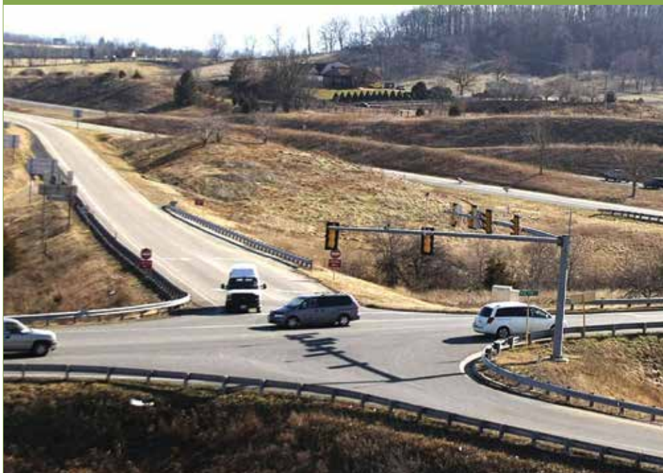
I-64 Access Ramps, Augusta County, Va.
