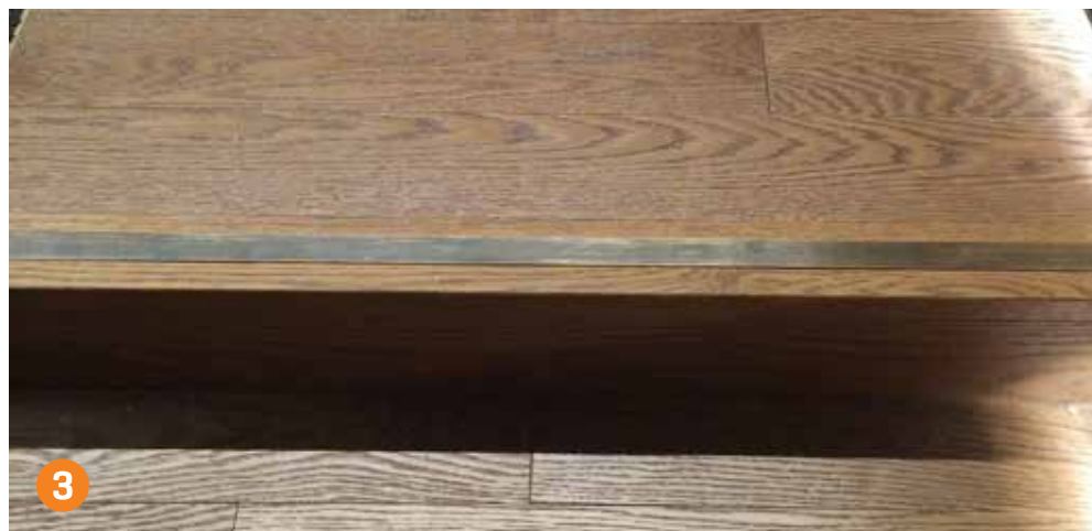
1) The field team drew a custom nosing using 3-D modeling software; 2) Our Virtual Design & Construction group printed the nosing in 3-D to serve as a mock up for review; 3) The 3-D model was sent to a local millworker to fabricate the custom nosing
