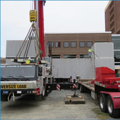
The existing generator, located outside of the South Patient Tower, was hoisted onto a low boy trailer and transported across campus.
