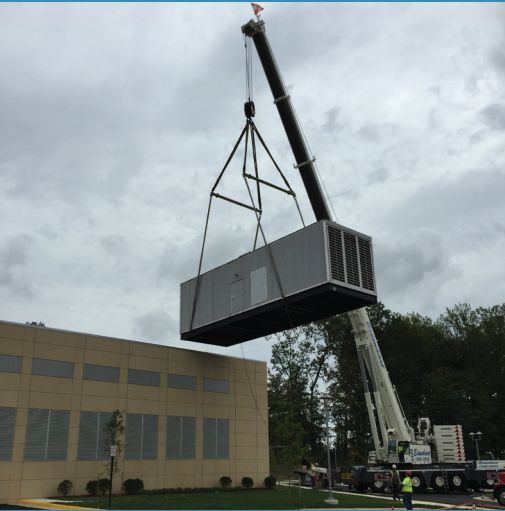
The generator arrived at the new CUP and was placed into its new home by a 250-ton crane.
