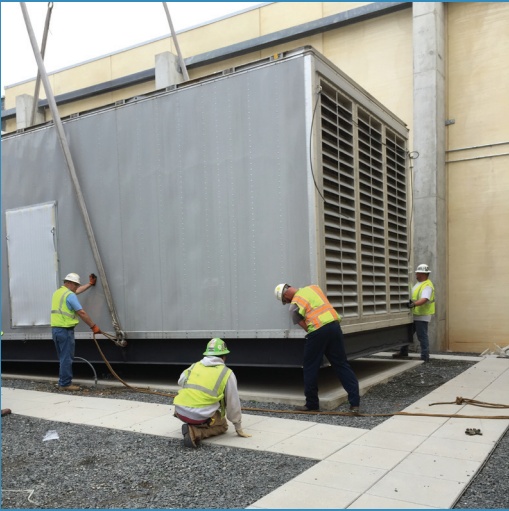
The generator was lowered into the CUP and guided into place by the electrical and rigging subcontractors.
