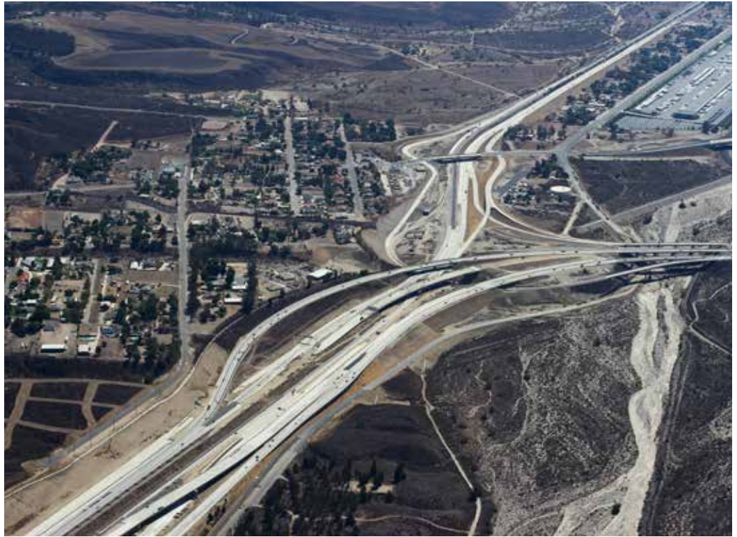
The Devore Interchange project improved safety and reduced traffic congestion by adding one new lane and two miles of truck bypass lanes in each direction.
