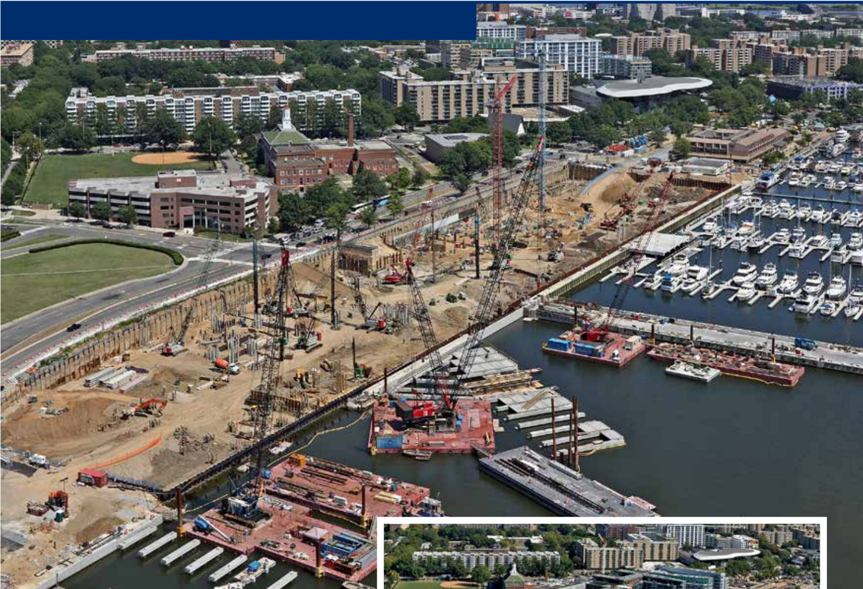
The Wharf, July 2015
