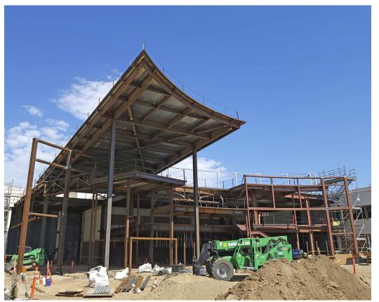
In June, Crews completed structural steel assembly on the new entrance to the Clovis Community Medical Center, which includes a curved canopy covering the main patient drop-off area.
