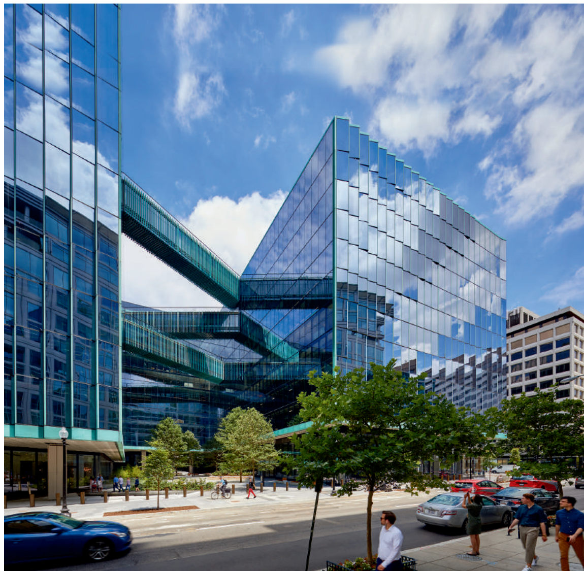
Midtown Center’s distinctive façade features a unique, patterned glass curtain wall with multiple elevations of 3D panels and pre-patinated copper cladding.
