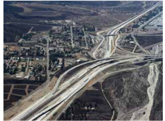
I-15/I-215 DEVORE INTERCHANGE MERIT WINNER DESIGN-BUILD CIVIL
