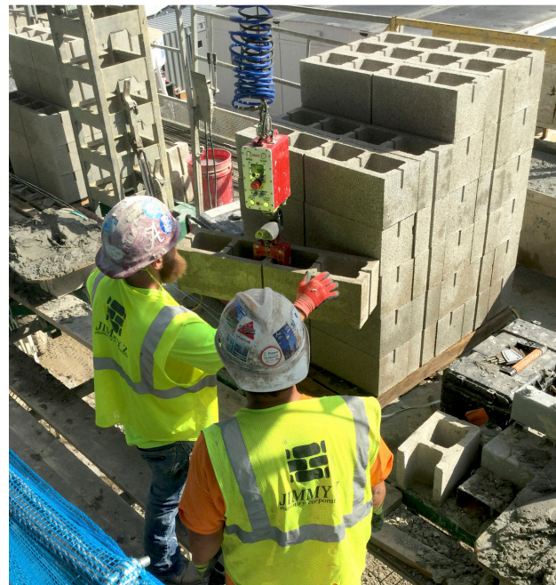
Masons place CMU blocks with assistance from the MULE, a mobile lift-enhancing unit designed to lessen the physical strain of this work.
