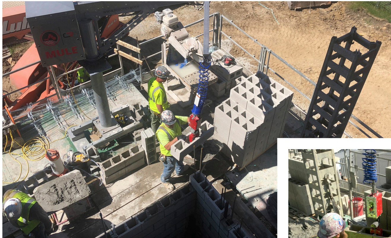
Masons place CMU blocks with assistance from the MULE, a mobile lift-enhancing unit designed to lessen the physical strain of this work.
