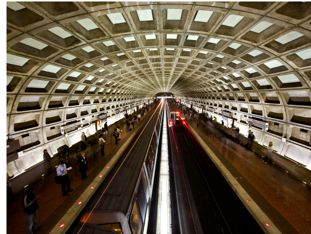
This page: C3M recently started work on their largest contract to date: a $52-million contract to upgrade electrical equipment in WMATA stations across Maryland, Virginia, and Washington, DC.
