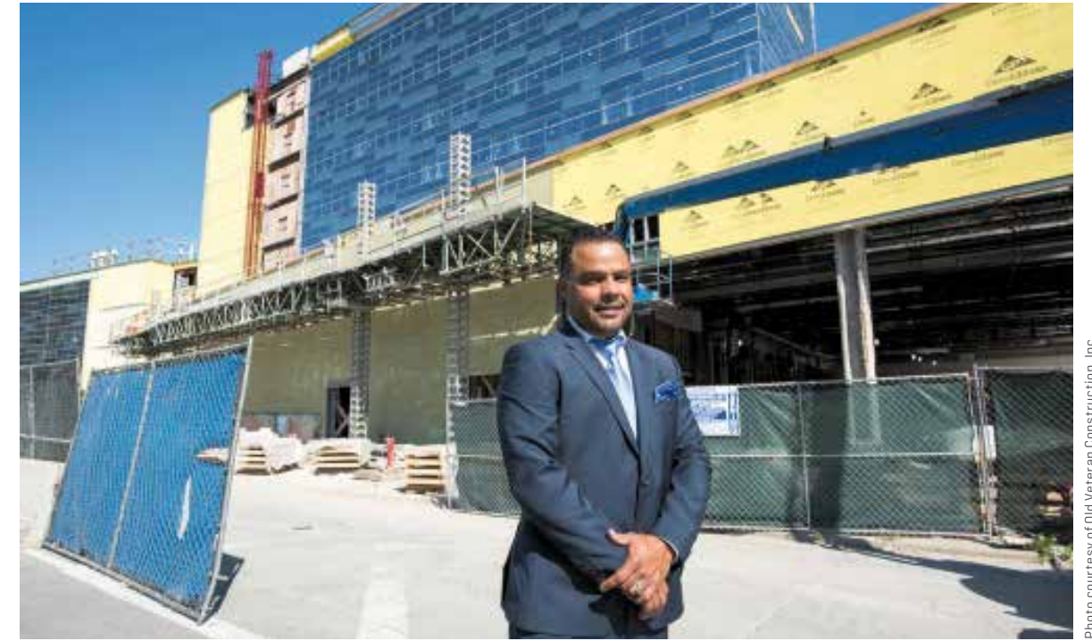
Photo courtesy of Old Veteran Construction, Inc.
