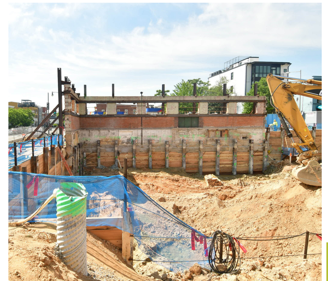
At the Harvard Substation, the new structure will be comprised of steel and concrete (pictured above). The project team demolished the entire structure except for the historical brick façade (pictured right).
