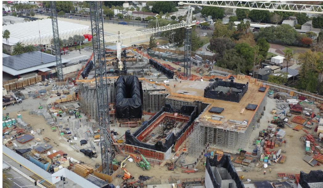
The team finished installing all base isolators at the end of 2022.
