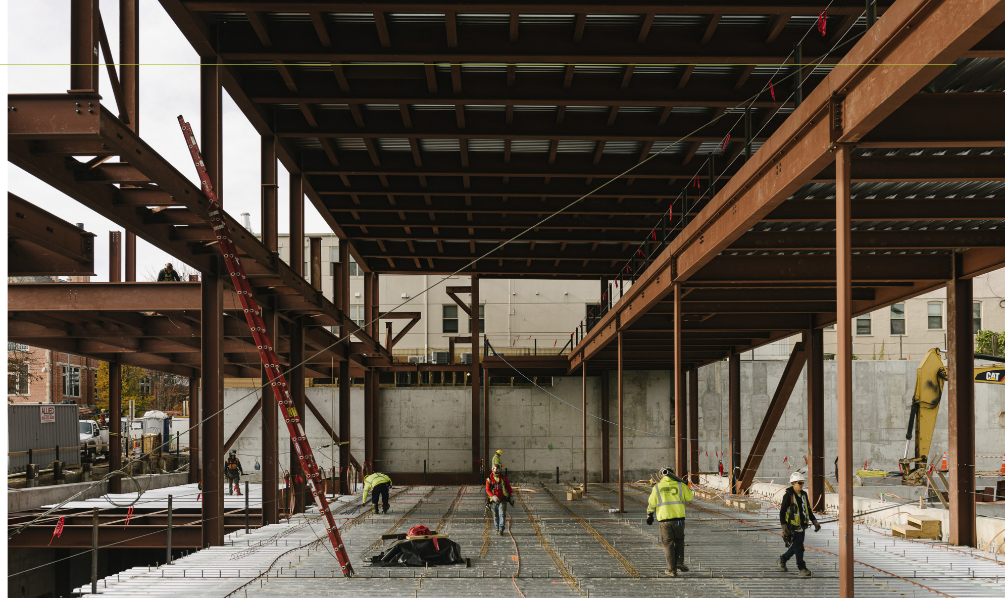
At the Harvard Substation, the new structure will be comprised of steel and concrete (pictured above). The project team demolished the entire structure except for the historical brick façade (pictured right).
